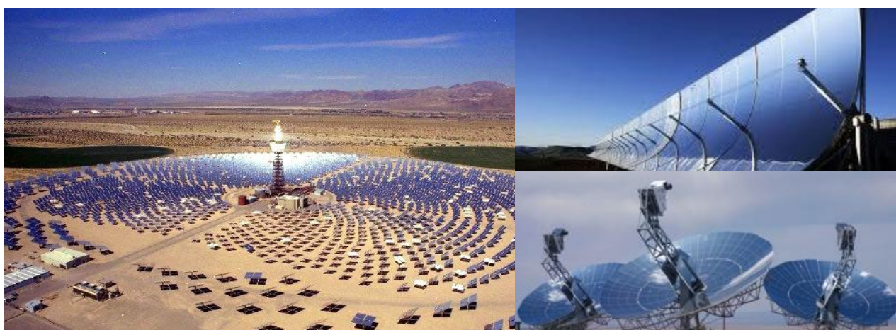
Figure 1. Layouts of concentrating solar mirror (parabolic dish from Sterling Energy Systems)
